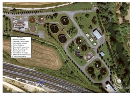
WWTP of Estella
